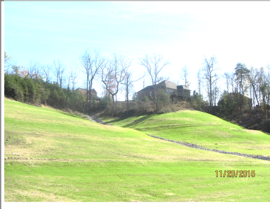
4. This is the same view as the above pictures with the Dangerous Highwall completely backfilled and revegetated.
